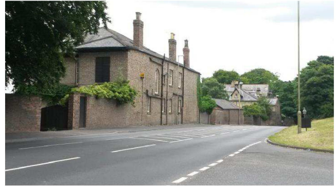
Use of traditional materials on approach to Malton town centre
