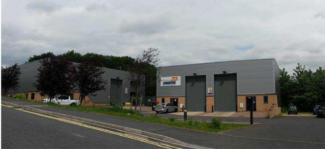
Existing business starter units on a neighbouring site, PPC cladding with brick at low level.
