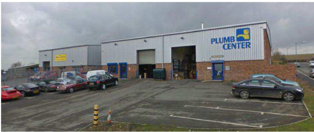
Existing business units on a neighbouring site, profiled aluminium cladding over brick at low level
